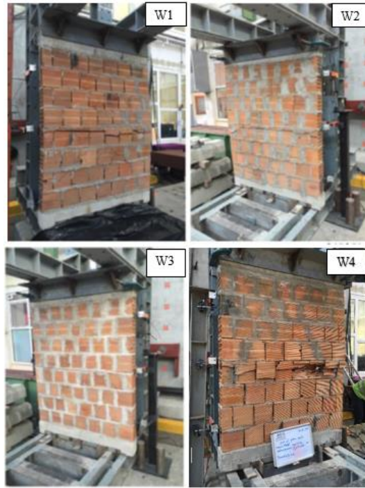
Figure 7. Crack propagation of each specimen at the end of the test. (Self-Elaboration).
