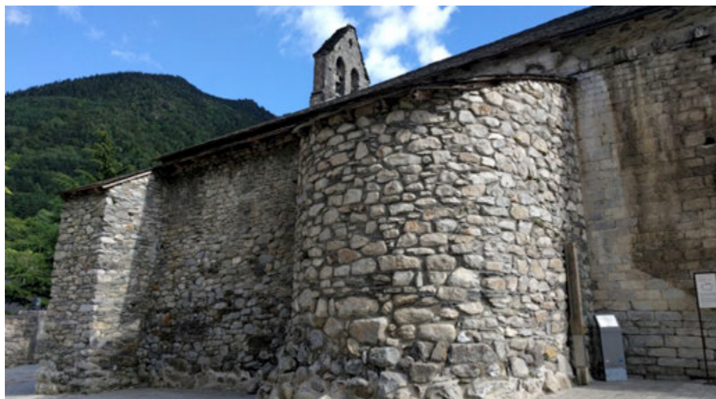
Figure 12. Counterforts of Santa Maria d'Arties, which produce passive thrust ( E_{pm} )
