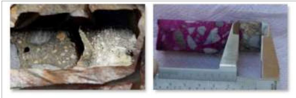
Figure 9. Carbonation Depth and Chloride Penetration
