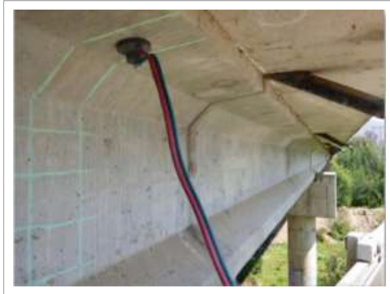
Figure 17. Air Permeability Measurement with PermeaTorr equipment on Prefabricated Beam Flange
