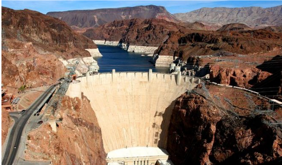
Figure 1. Hoover Dam in the US. Example of large exempt infrastructure
